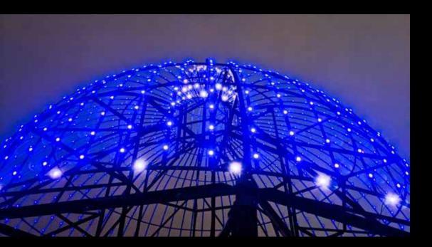
On Aug. 10, 2013, Borisch decided to restore the historical dome on top of McKay Tower, replacing the screw-in incandescent bulbs with roughly 1,200 small LEDs capable of glowing in a variety of colors and patterns as well as producing multiple color-changing effects and animated images.
